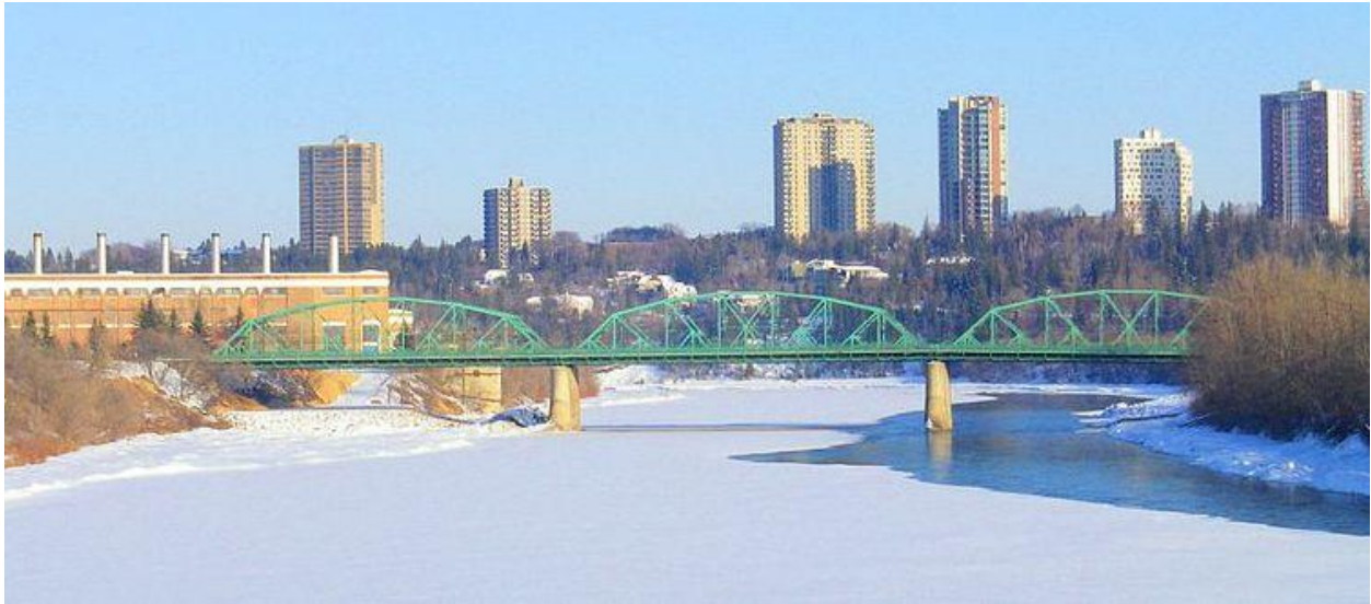
Existing Walterdale Bridge
